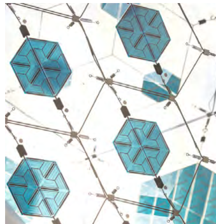
Hexagonal organic photovoltaic modules Produced by OPVIUS and installed at the German Pavilion at the 2015 EXPO Milano. Photo by LAPP Group.
